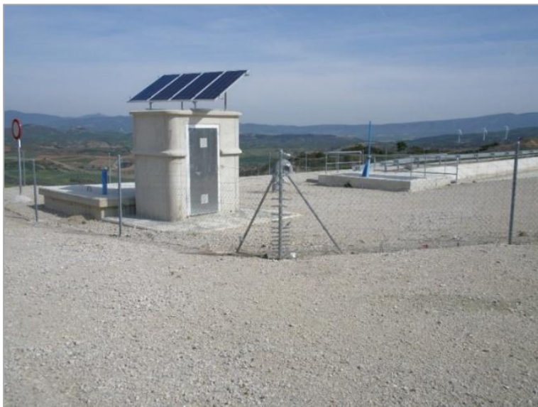
Figure 27 Solar panel on irrigation station, Source: INTIA
