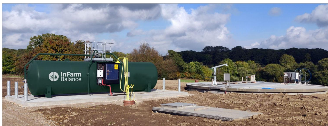
Figure 7 Acidification of manure. InFarm Balance NH4+. source: Infarm Solutions A/S
